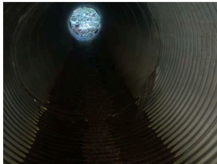
Coupled connection. Fabric sticking through
